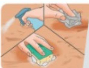
Clean the surface and remove any dust, unsound or contaminated material, plaster, oil, paint, grease, corrosion deposits or algae.
