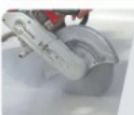
Saw cut the concrete areas to a square or rectangular profile to a minimum 10mm depth at the extreme edges. Roughen the surface free of loose particles and dust and saturate with water. Remove excess/standing water.
